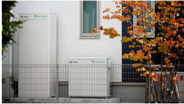
Ene-Farm - 1kW-NG. Japan Ene-Field. 0.7-2.5 kW-GN/Biogas-EU
