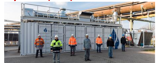
High-Temperature Electrolyser (HTE) Salzgitter Flachstahl GmbH. SOEC 720 kW 200 Nm 3 o 18 kg H 2 /h GrInHy2.0 project Electrical efficiency 84 % (LHV)-2022
